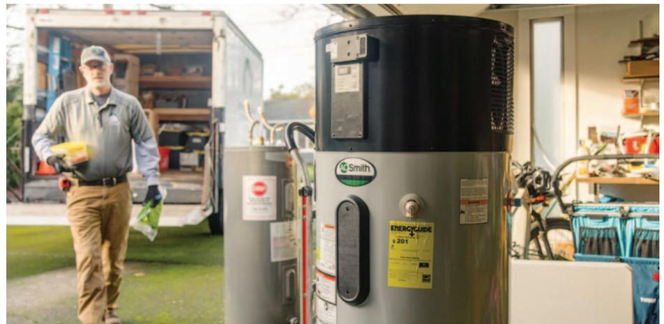
*Smart heat pump water heaters are equipped with automation features that help you use less energy. Photograph provided by Northwest Energy Efficiency Alliance*
